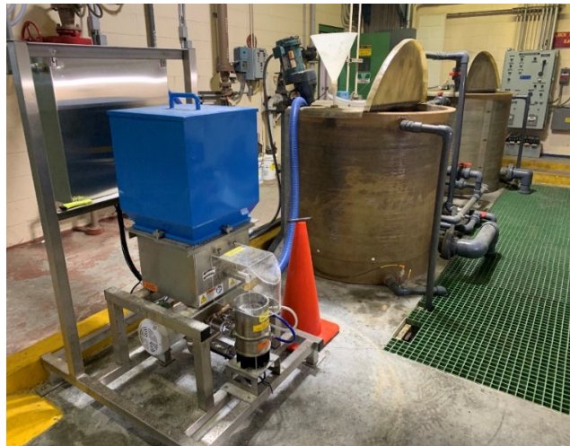
Figure 4-17 – Polymer Feed System
