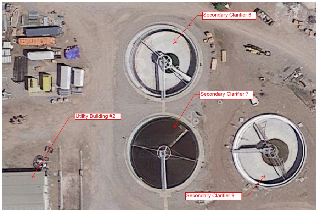
Figure 4-7 – Secondary Clarifiers 6 through 8
