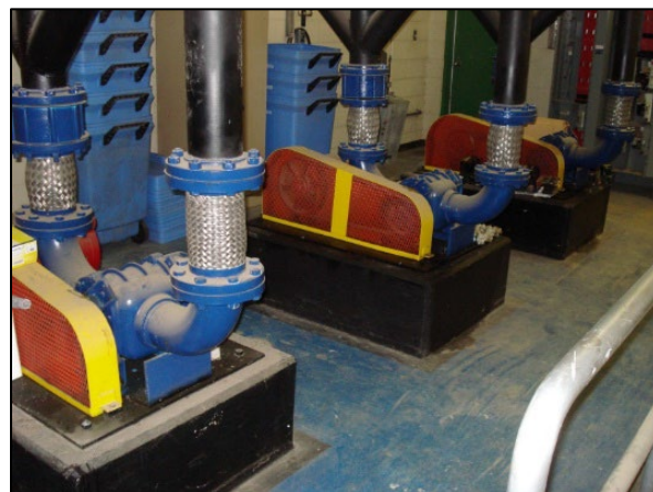
Figure 4-14 – UB1 Blowers (Tank 1)
