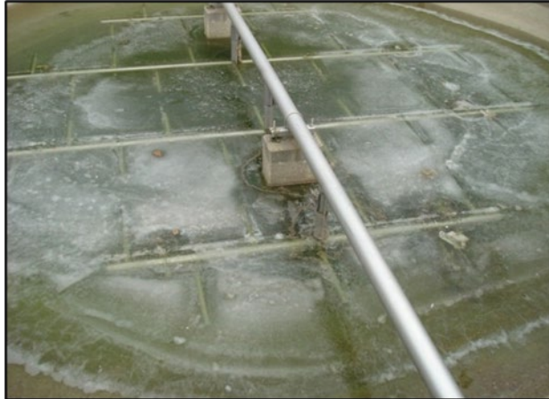
Figure 4-13 – Sludge Storage Tank 2
