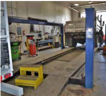
FIGURE 42. UNDERSIZED FLEET SHOP
