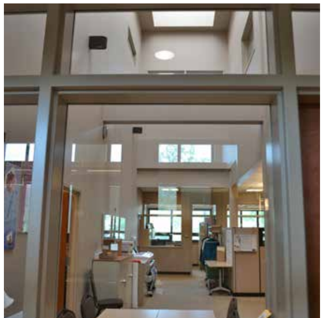
FIGURE 91. LIGHT WELLS DAYLIGHT TO BUILDING INTERIOR
