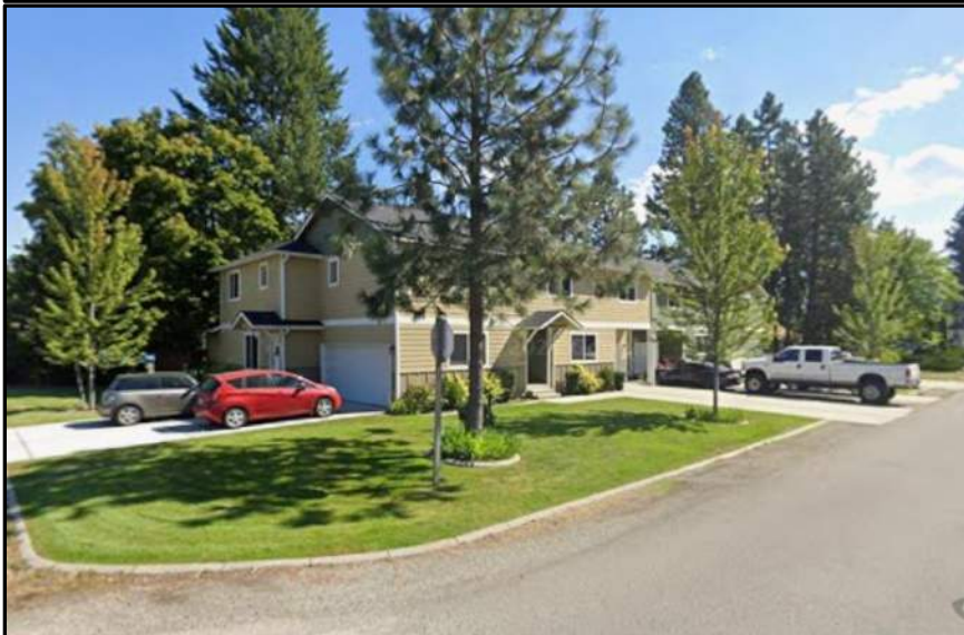
Looking south from N Catherine St at Swaboda Estates Twin Homes
