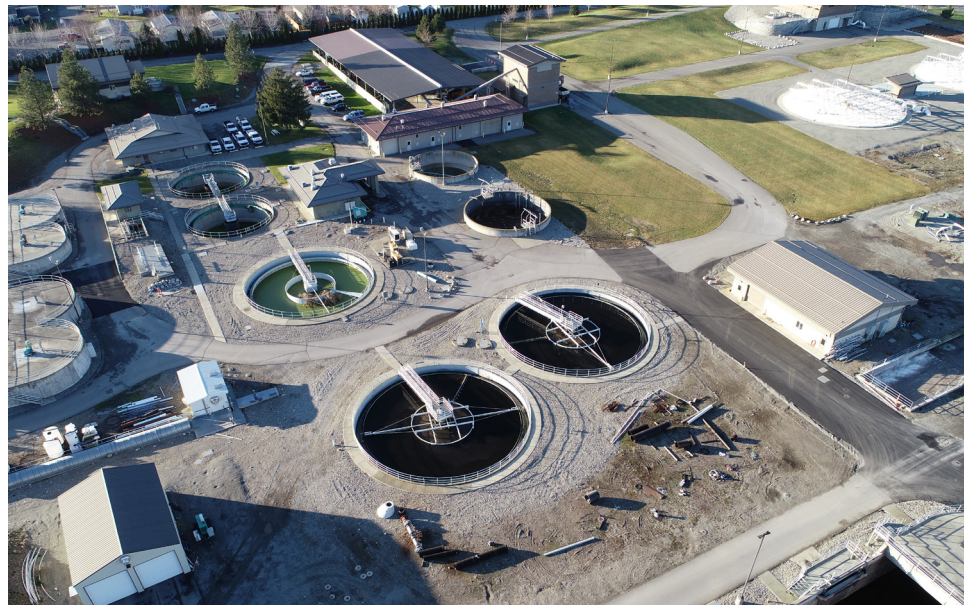
Post Falls WRF Solids Process Facilities, June 2024.
