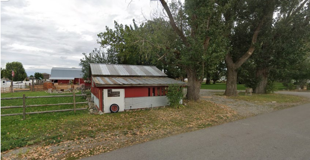
Looking East from Guy Road at northwest boundary
