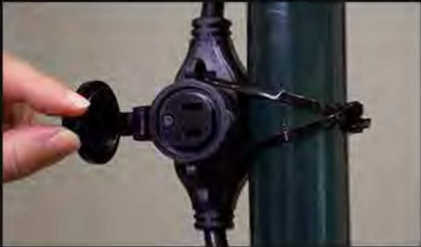
Capped and gasketed plug receptacles to shield water from electrical contacts.
